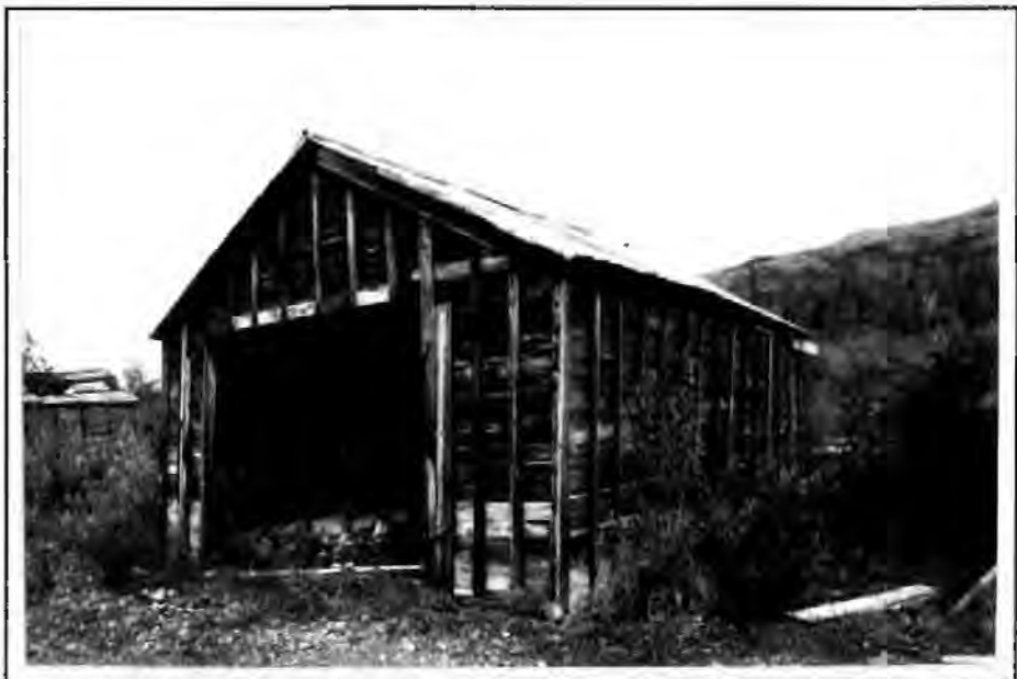
Figure 166. The Garage at the Fullerton Camp, 1993. The view is looking northeast.
